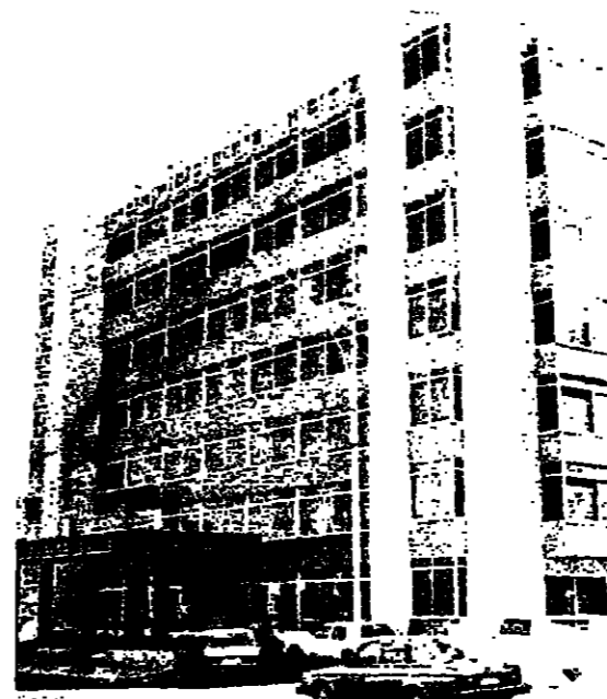
Front elevation of Commodore Hotel.
